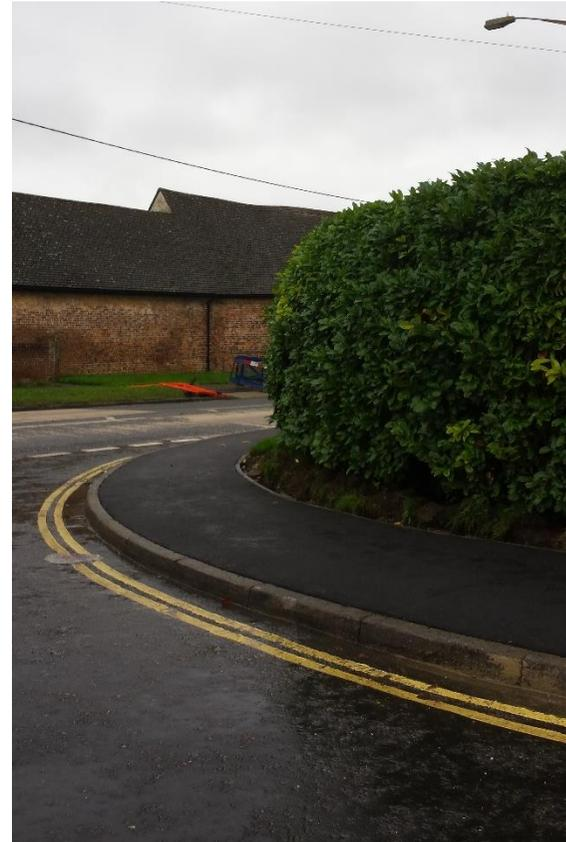
A small section of new footway was installed on the corner of The Street and Hatfield Forest Road where previously there was no drop kerbs to facilitate pedestrians crossing at this point
