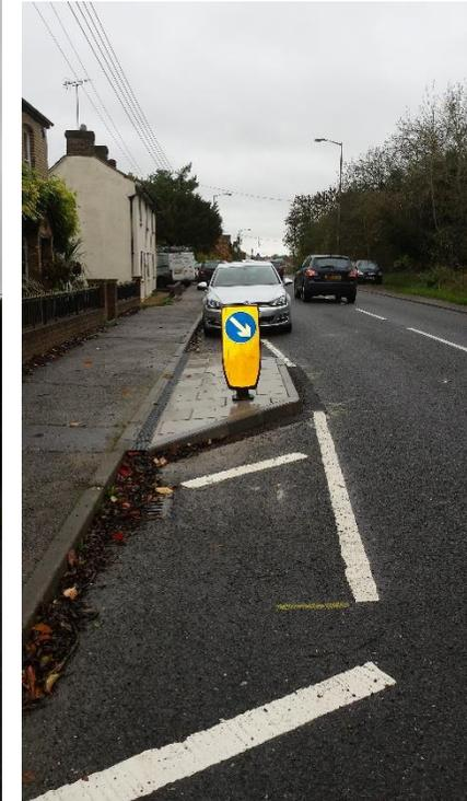
A series of build outs and refuges have been installed throughout The Street for a distance of approximately 1 mile
