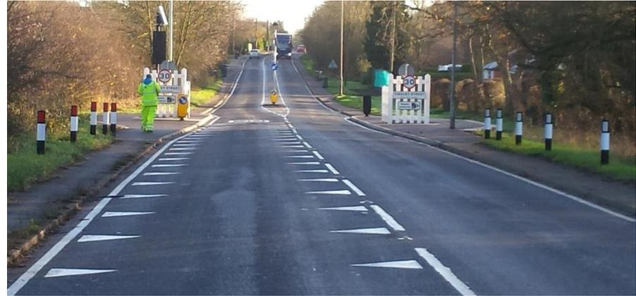
The existing gateway feature was replaced with a new low maintenance structure with the kerbline built out and dragons teeth installed to create the impression of the road narrowing as you enter Takeley from the M11 side.
